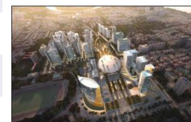
Yangon Central Railways Station, Myanmar
